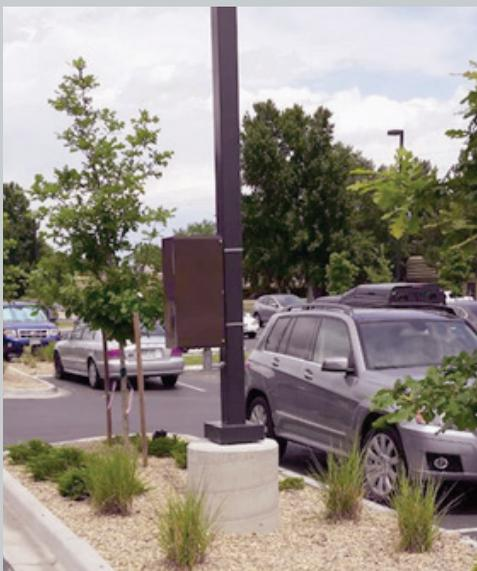
*Painted Power Extenders blend with the light pole for a more aesthetically pleasing solution. Radios are located at the top of the pole.*
