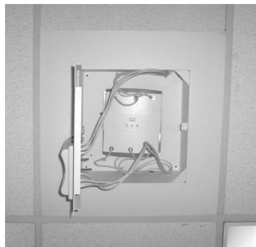
24x24x8 MIMO Ceiling Tile Enclosure – Installed in Ceiling Tile Grid Displayed with a TerraWave 802.11n Dual Band 2.4/5 GHz 2.5/4.5 dBi Ceiling Mount MIMO Omni Antenna and a Cisco 1252 Access Point
