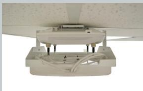
Denault chose to mount many of the APs and antennas using a Co-locating Mount that articulates +/- 25 degrees, to enable precise positioning of the beam.
