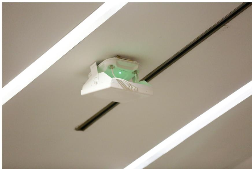
Co-Locating Mounts with access points and antennas were installed in front of the auditorium.
