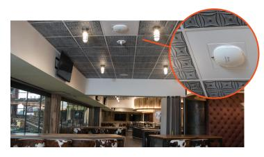
In the suites and other interior parts of the stadium, Ventev recommended using the Ceiling Tile Enclosure with Interchangeable Door for an inconspicuous solution to deploy access points in a suspended ceiling tile grid. The lightweight enclosure reduces strain on ceiling grid, enables access points to be serviced without removing the entire enclosure, and blends seamlessly into the environment.
