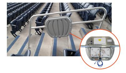
Ventev's handrail enclosures were installed in 200 locations throughout the stadium. After the challenges of retrofitting the stadium for the upgraded network, the KLA team was pleased that the installation of the handrail enclosure was simple and straightforward.
