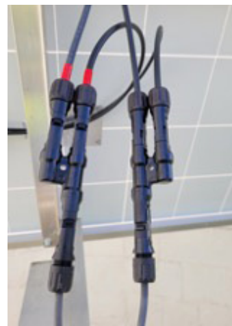
FIGURE 11: Two Module Mount with Module Interconnect Connectors
